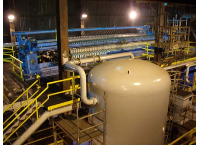
Filter Project: Construction Near Completion
